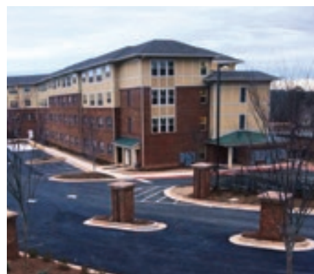
The Fifth Third Community Development Corporation invested $7.8 million in the Panola Gardens project in Lithonia, Georgia, in 2014. The 85-unit apartment complex is designed for seniors and the spaces will be occupied by residents who are at or below 60 percent of the area median income.
